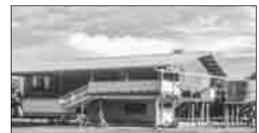
Staff house for Bolave Sub Health Center, funded by National Government through Hon. Timothy Masiu initiative projects approved by the Southern Region DDA Board.
